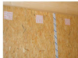
Right: Picture four – Internal view of pre-fab wall panels with joints and insulation holes taped and sealed for air-tightness
