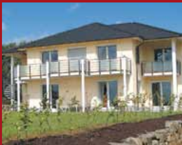
Single-family house | Photo: T. Weber
