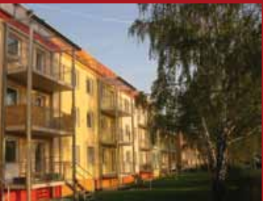
Retrofit | Photo: PHI
